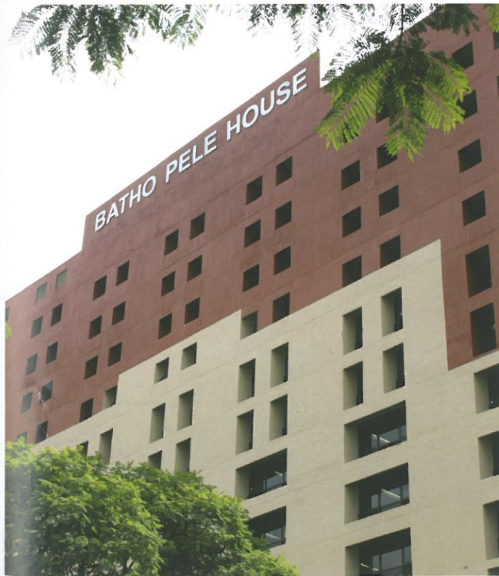
The windows of the building are recessed to limit the amount of sunlight and warmth that enters the offices.
